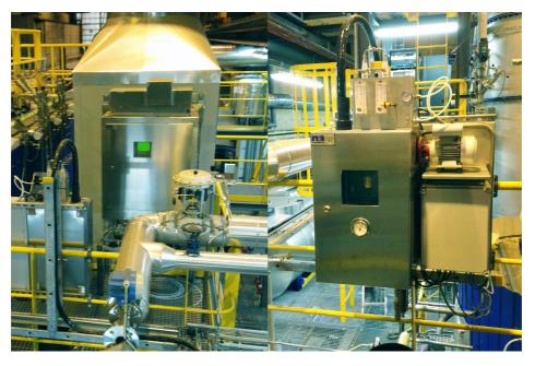
Figure 8: On the left a gas analyzer from Norsk Analyse A/S, on the right a gas conditioner also from Norsk Analyse A/S<sup>16</sup>
